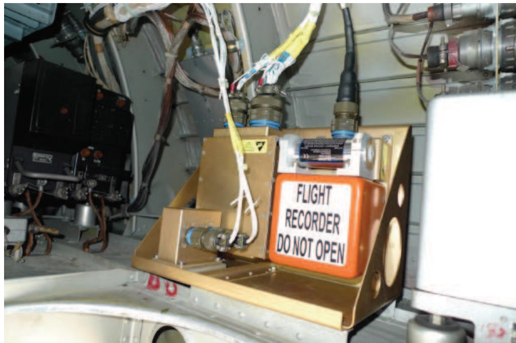
Picture of installation
